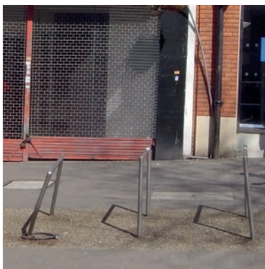
Existing cycle stands are in poor condition
