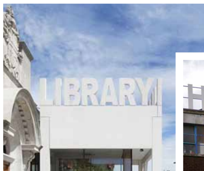
Thornton Heath Library by FAT Architecture
