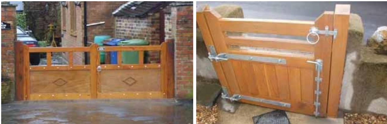
Figure 9-3 Example of flood gates
