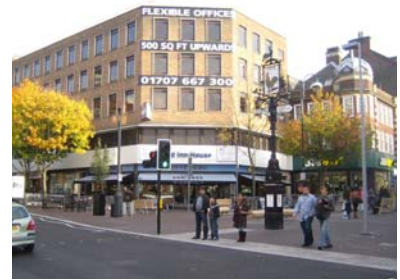
5-storey at no. 2 Carshalton Road and 3-storey building with domed roof on the site of the Cock Hotel
