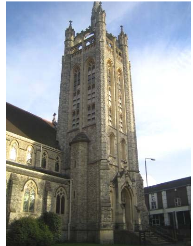
Trinity Methodist Church tower
