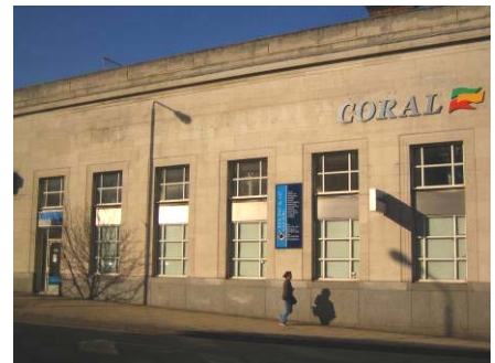
The Coral building, no. 17 High Street
