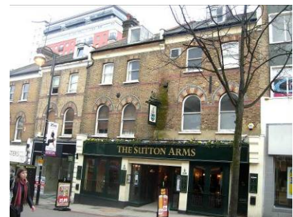
Terrace with original sash windows and brick detailing. The dormer windows are visible.
