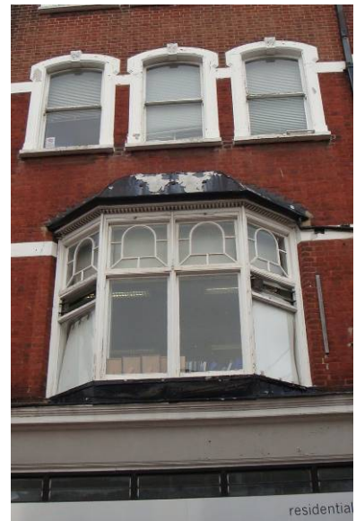
Original canted window with glazing bars at 32-34 High Street
