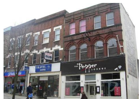
No. 67 High Street, now the end building in the terrace.
