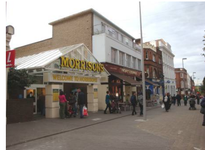
New buildings at 31-35 High Street interrupting the historic High Street
