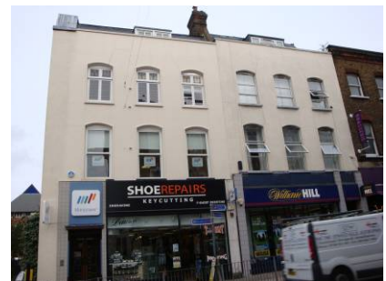
Painted brickwork at nos. 14-18 High Street
