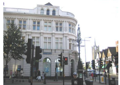
Locally listed Barclays Bank building
