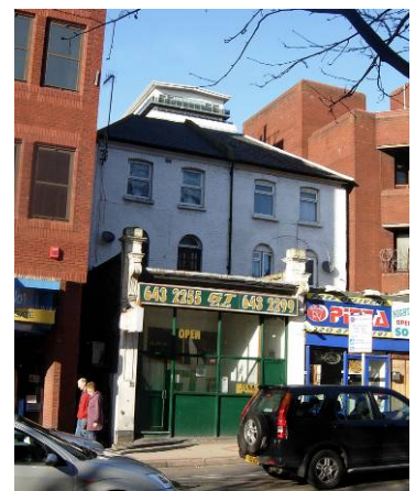
Nos. 7-9 Carshalton Road
