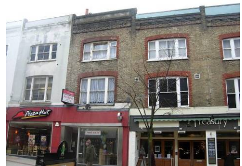
Four of the terrace at 51-61 High Street. The buildings to the right are not painted and the original detailing is visible.
