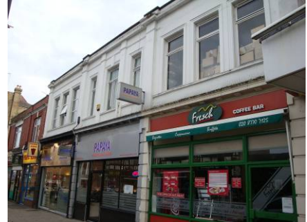
Two-storey shops at nos. 1-9 Cheam Road.
